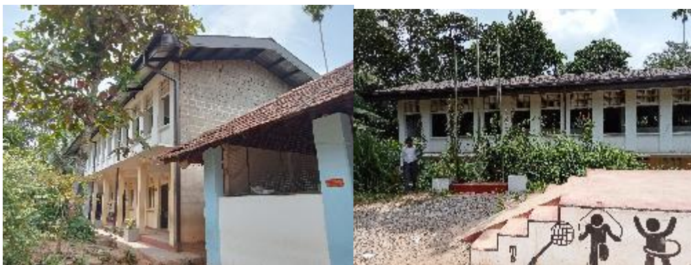
Figure 13 Catchment roof, and location for the tank
