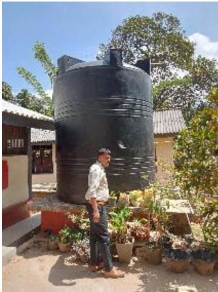
Figure 4 Large Tank to Store Pradeshiya Sabh pipe Water
