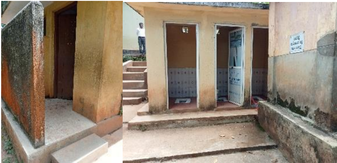
Figure 14 Just two toilet units with cover wall, other units with no wall not suitable for girls
